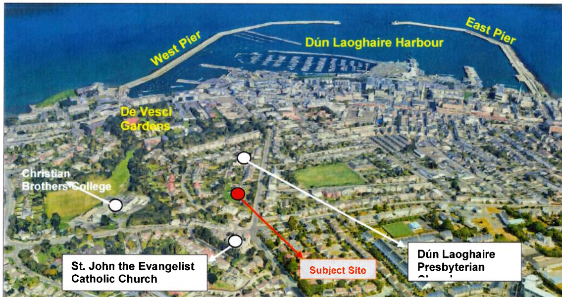
Figure 3.0 Aerial image showing the context surrounding the subject site
