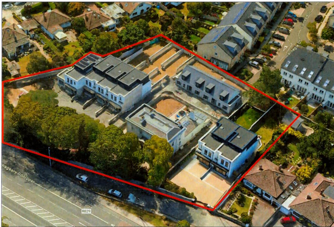
Figure 43.0 Satellite view of the development granted under ABP. Ref. 303601.
